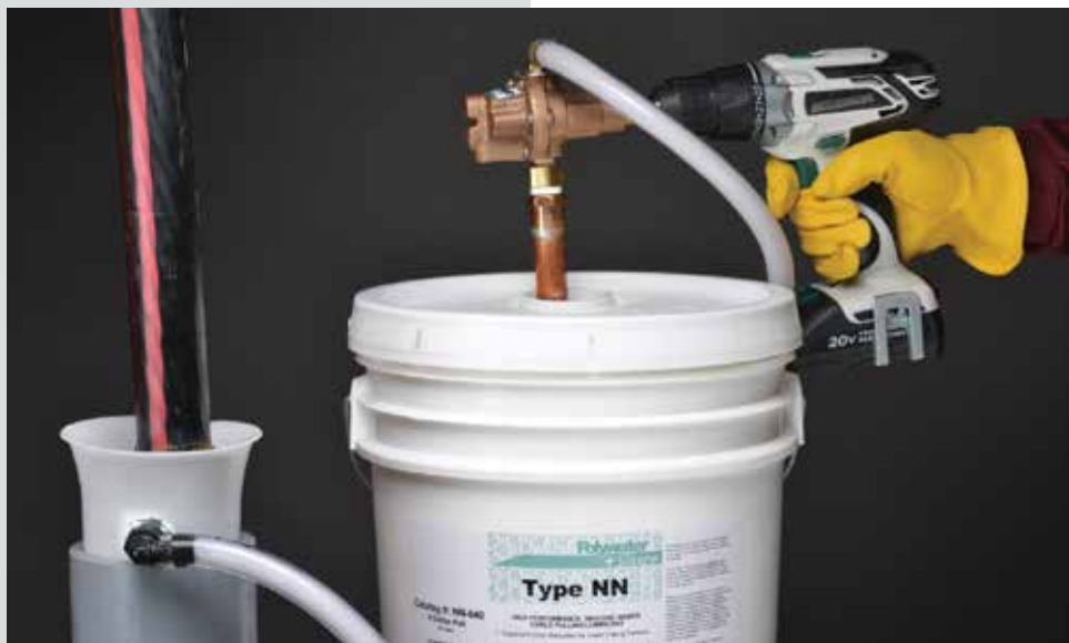
Polywater + Silicone lube is easily pumped
