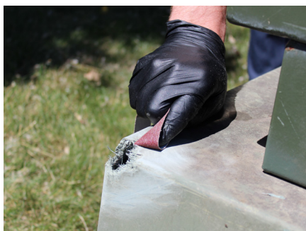
Clean and sand before applying BRK
