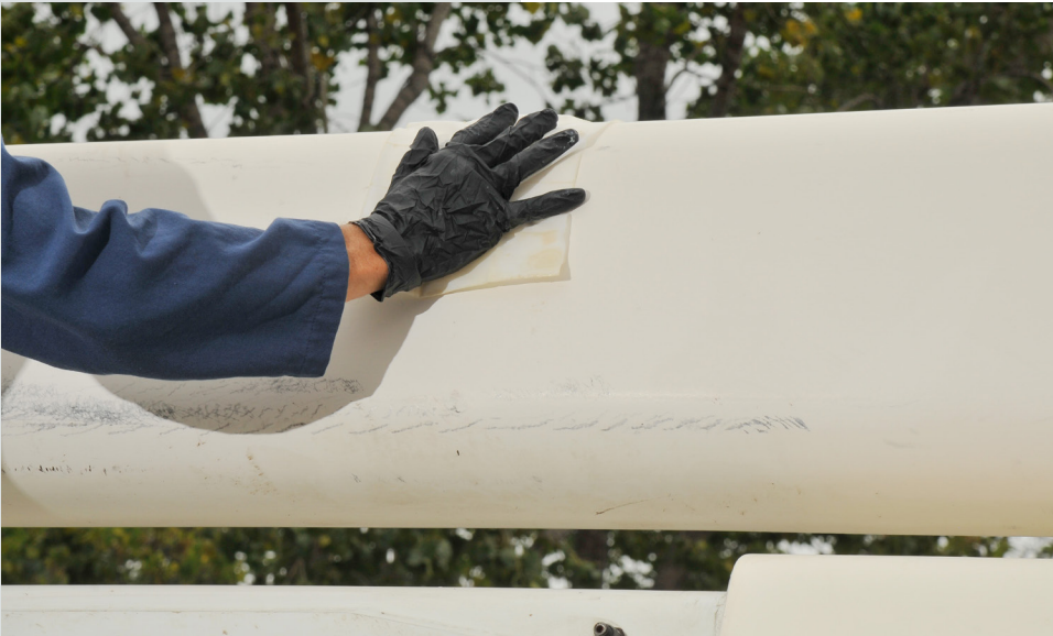
Waxing protects the gel coat
