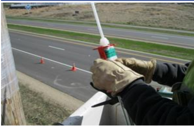
Insert cartridge into high-ratio caulking tool
