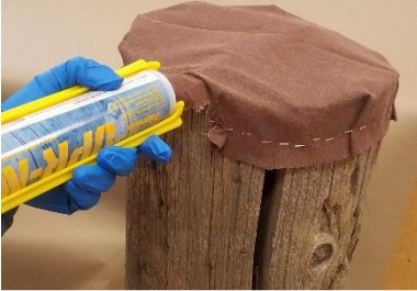
Inject UPR-NF on top of pole. Move static mixer tip while injecting.
