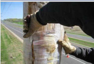
Cover injection port with stretch wrap
