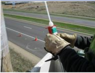
Insert cartridge into high-ratio caulking tool
