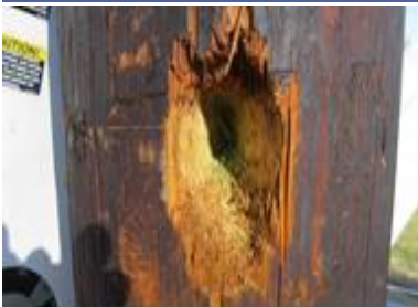
Remove all debris and water from the hole
