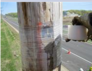
Wrap hole with stretch wrap
