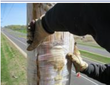
Cover injection port with stretch wrap
