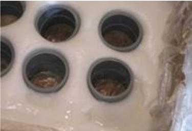
8. Mix and install each InstaGrout kit individually, waiting for each kit to react before deploying the next kit (approximately 20 minutes). InstaGrout bonds well to itself so that multiple applications have the same strength as a single deployment of InstaGrout.
