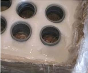
8. Mix and install each InstaGrout kit individually, waiting for each kit to react before deploying the next kit (approximately 20 minutes). InstaGrout bonds well to itself so that multiple applications have the same strength as a single deployment of InstaGrout.
