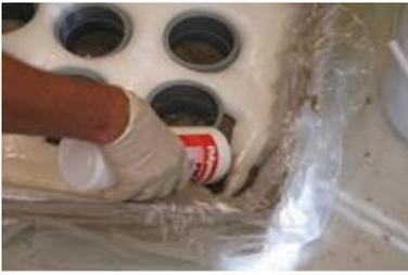
7. Inspect seal to make sure InstaGrout adheres to all component edges and surfaces so that no gaps are apparent.
