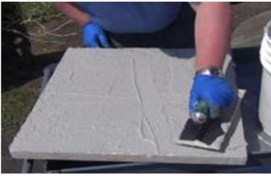
8. Working life at 72°F (22°C) is about 2 hours. Set time is about 4 hours and functional cure time is about 24 hours. Dura-Plate 100 cure times are dependent on temperature. Higher temperatures shorten these times. Lower temperatures lengthen these times.
