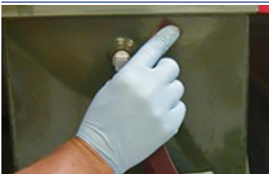
Sand or brush repair area
