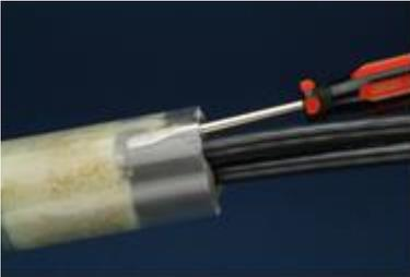
9. After sealant has fully set and cured, use a screwdriver to check for voids in the FSTBP Seal. Foam seal should be solid throughout the duct. If any holes or voids are detected in the inspection, use a screwdriver to cut into top of foam and enlarge a path for new material. Inject additional sealant directly into the void area.
