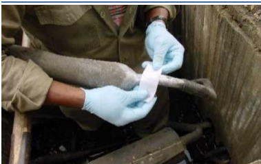
Cleaning cable with cleaning wipe
