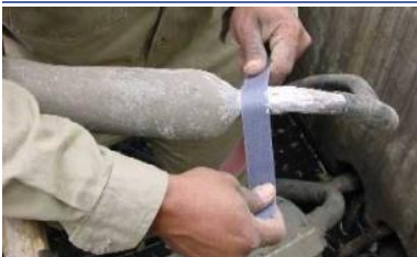
Sanding cable for repair
