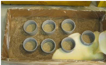
PedFloor is mixed and poured
