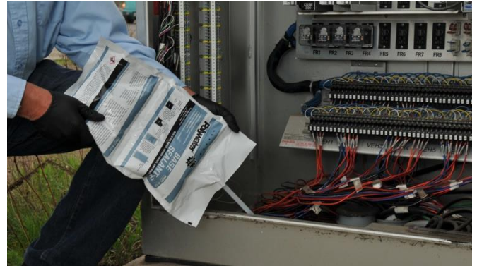
PedFloor repairs and creates a barrier for cabinet bases.
