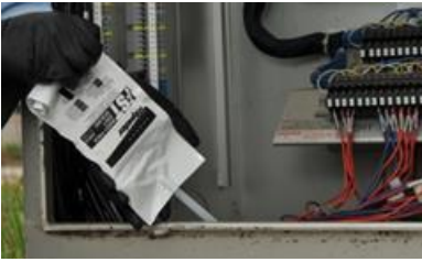
Fill gaps with FSTBP
