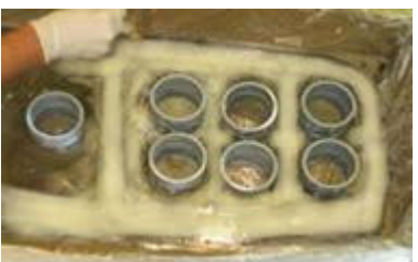
Spread PedFloor with stick
