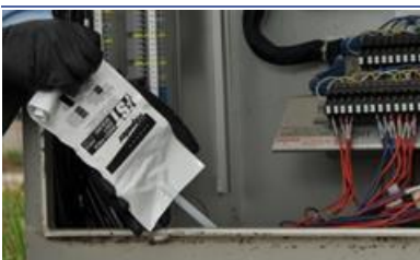
Fill gaps with FSTBP
