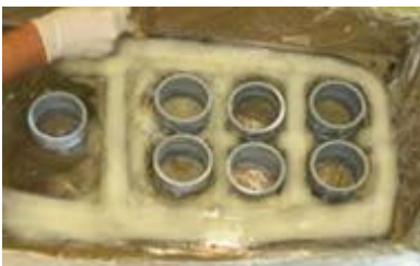
Spread the PedFloor material with stir stick
