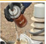
Type RP<sup>™</sup> Fast evaporating cable cleaner Type FD<sup>™</sup> Fast-drying multipurpose industrial and maintenance cleaner
