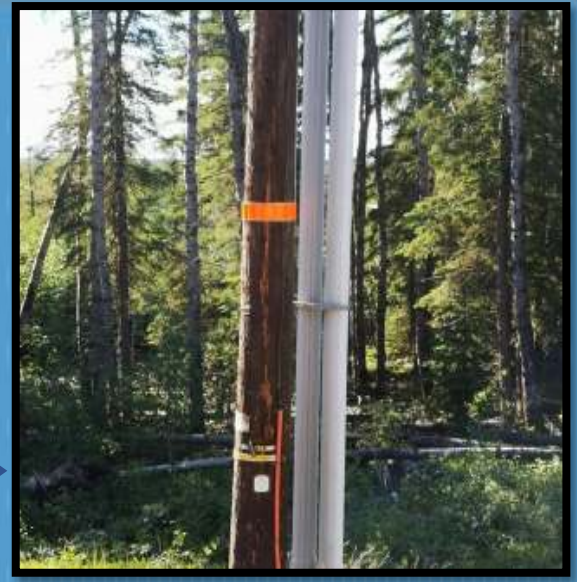
Close up of cracks
