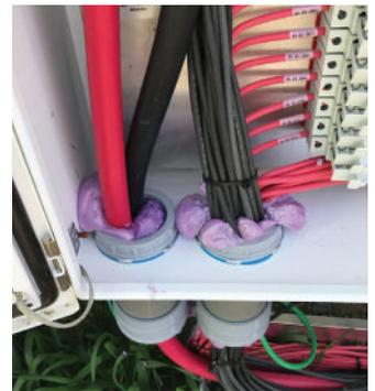
Polywater AFT can be used to seal more than conduits, including solar inverters, riser poles, U-Guards, raceway entrances, and more.
