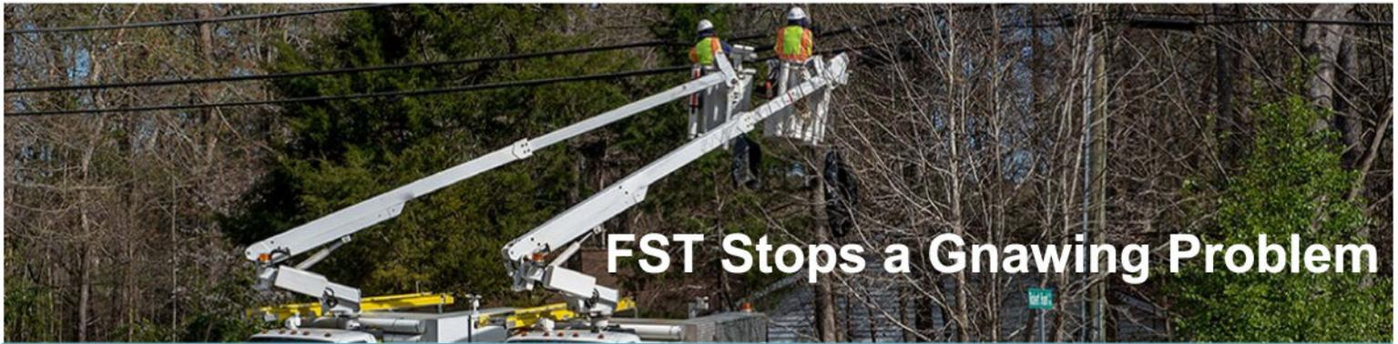
Risers Sealed with Polywater FST to Stop Squirrels from Damaging Cables.
