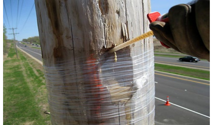
Polywater UPR PR Pole Repair can be applied without drilling extra holes into the pole.
