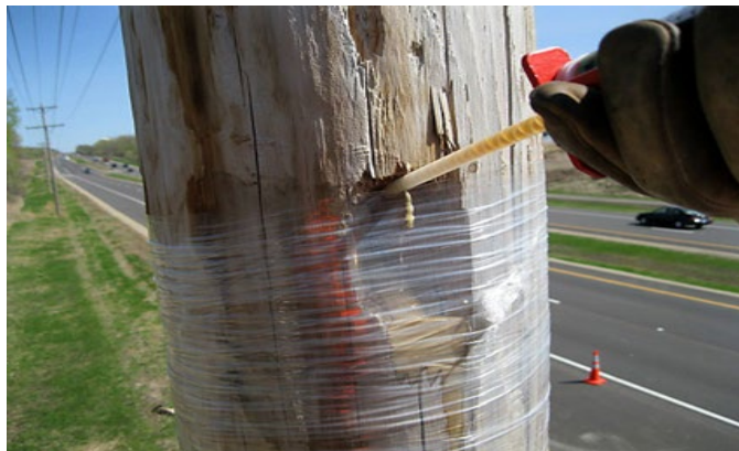
Polywater UPR NF Pole Repair can be applied without drilling extra holes into the pole.
