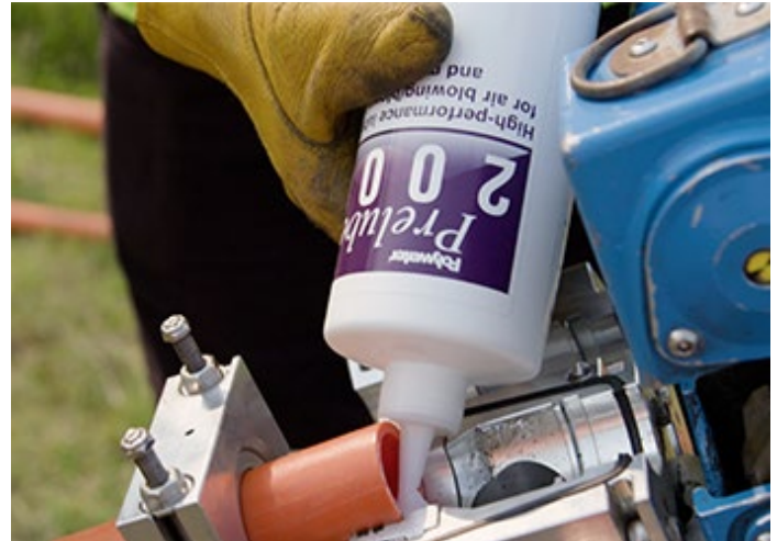
Prelube 2000 applied to duct prior to blowing fiber cable
