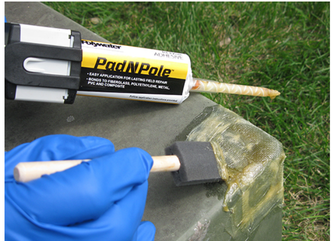
Polywater Pad N Pole is used to repair damaged enclosures.
