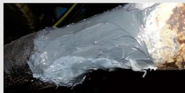
**A closer look at the repair process to create a flexible seal.**
