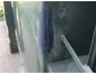
Completed repair with Polywater PowerPatch.
