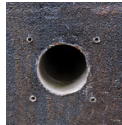
Core drill and pilot holes.
