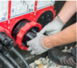
Inserting a PHSI-150-D3 into a Varia.
