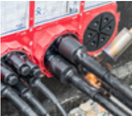
Applying heat to the heat shrink.
