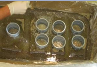
Spread the PedFloor material with stir stick
