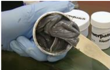
Mix 2-part paste sealant to a uniform grey color
