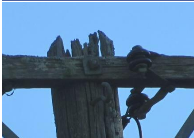
Remove all debris.
