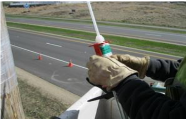
Insert cartridge into high-ratio caulking tool
