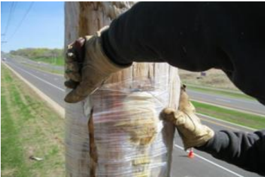
Cover injection port with stretch wrap
