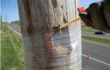
Insert static mixer and rapidly inject material into hole
