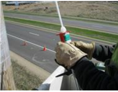
Insert cartridge into high-ratio caulking tool
