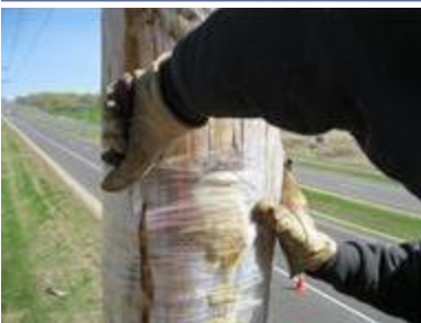
Cover injection port with stretch wrap
