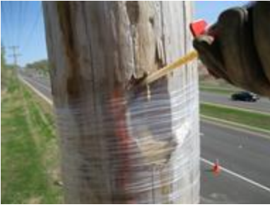
Insert static mixer and rapidly inject material into hole
