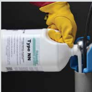
Pouring lube into a conduit stub-up
