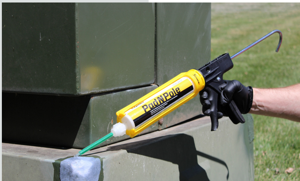
Finished Pad N Pole repair
