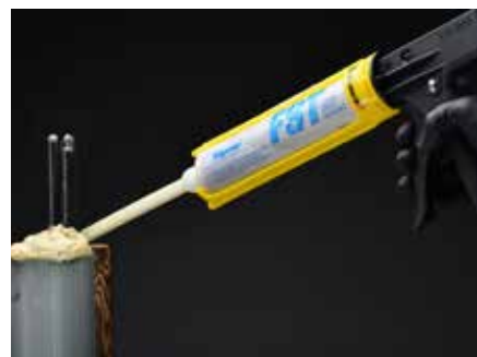
Riser seal application
