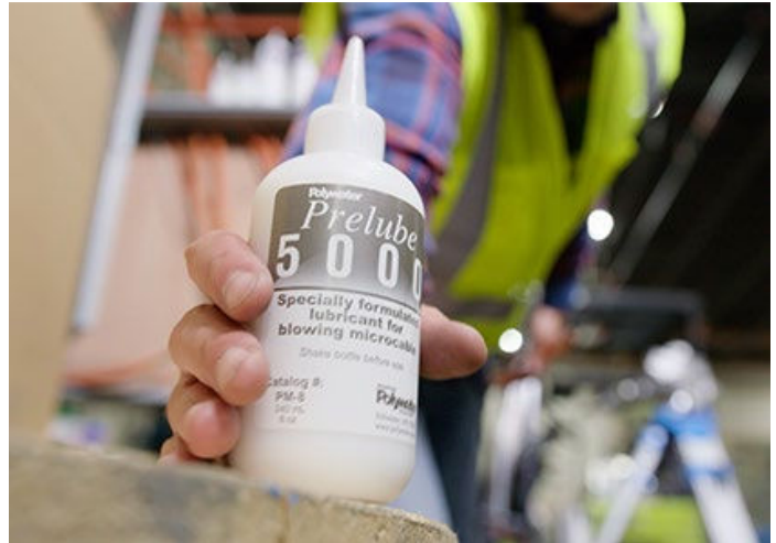
Prelube 5000 applied to duct prior to blowing fiber cable
