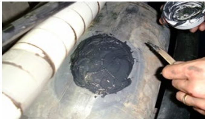
The AirRepair Leak Repair System seals air leaks in pressurized cables and splices.
