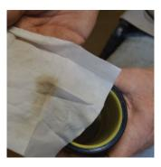
Effectively removes contaminants prior to electrofusion.
