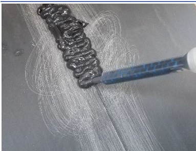
Apply PowerPatch
