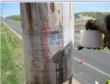
Wrap hole with stretch wrap
