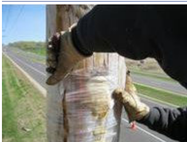
Cover injection port with stretch wrap
