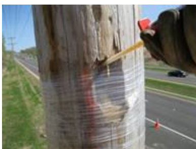
Insert static mixer and rapidly inject material into hole
