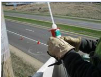
Insert cartridge into high-ratio caulking tool
