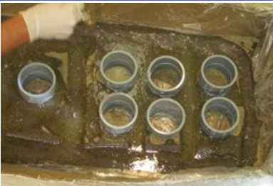
Spread the PedFloor material with stir stick
