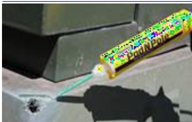
Applying thin coat of Pad N Pole
