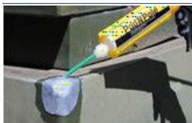
Coating fabric with Pad N Pole
