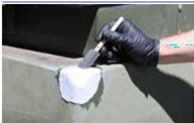
Attaching fabric to enclosure
