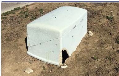
Large holes need backing
