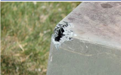
Enclosure damage
