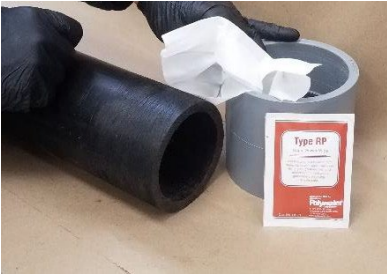
Clean Coupling and Conduit with Cleaning Wipe
