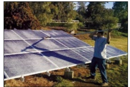
SPW™ being used to clean panels.
