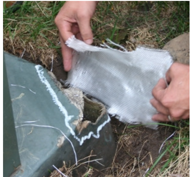
Fiberglass cloth saturated with the high-strength, two-part resin makes the permanent PowerPatch® Pad N Pole™ Repair.
