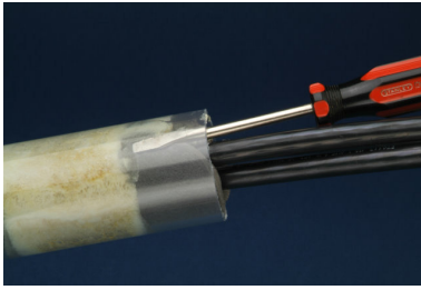
Using screw drive to check for voids
