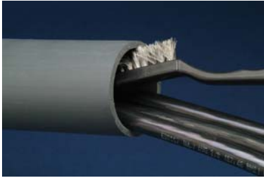
Clean duct with wire brush, solvent wipe.
