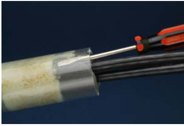
Using screw drive to check for voids
