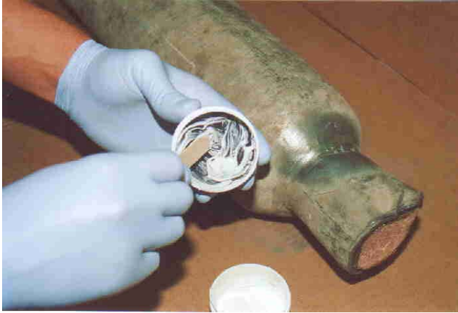
Photo 1 Mixing AirRepair® Paste
